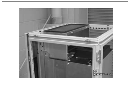
3.46: Top duct installed
