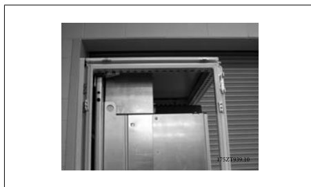
3.38: Top duct work and enclosure top installed
