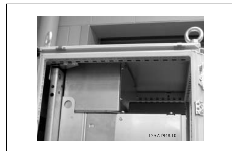
3.49: Enclosure top installed
