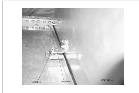
3.58: Move mounting screws from the outer hole to the inner hole
