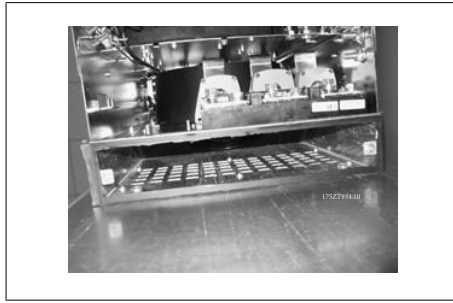
3.33: Bottom duct adapter installed
