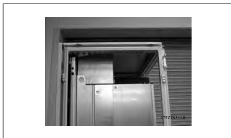
3.38: Top duct work and enclosure top installed
