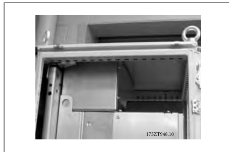
3.49: Enclosure top installed
