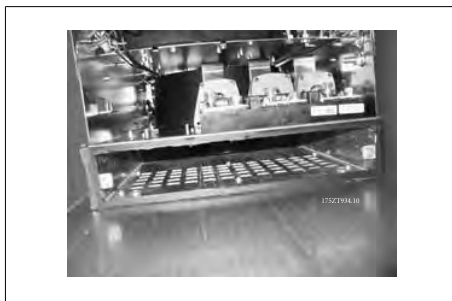
3.33: Bottom duct adapter installed
