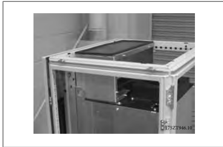
3.46: Top duct installed
