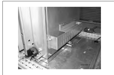
3.59: Bottom duct installed.
